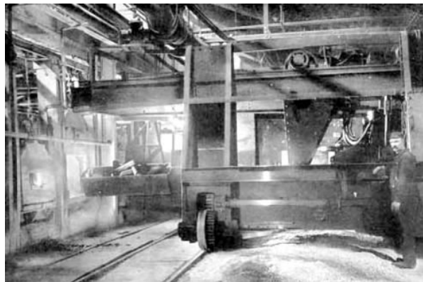
Charging a Siemens-Martin furnace
