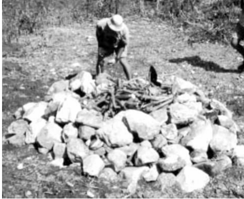
Building a working lime kiln
