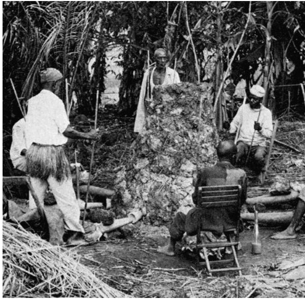
Haya smelter in 1977. Note the 8 (leaky) tuyeres!
