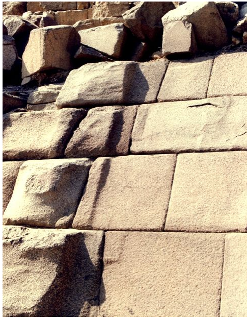
Partially polished granite blocks around the entrance to Menkaure's pyramid at Ghiza, Egypt
