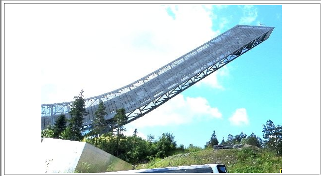
"Holmenkollen" ski jump construction in Oslo, Norway
